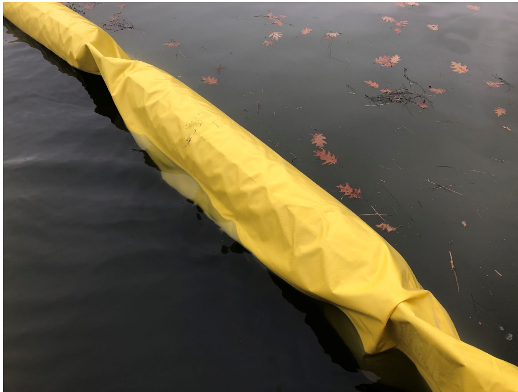
Offshore apex (yellow segment) of turbidity barrier deployed on western diver burial work location. Inside the barrier is evident by leaves and turbidity water (at surface).
