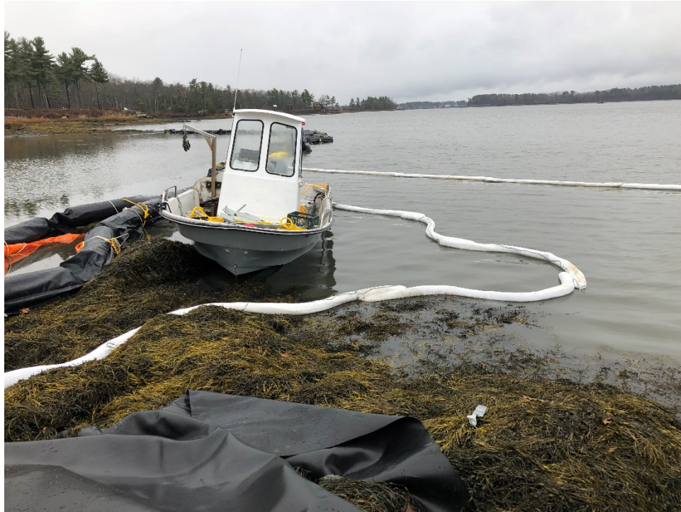
Mackworth Env vessel upright and on rocks at Durham landing. Absorbent booms deployed by Durocher. Turbidity barrier meant for the eastern diver burial operation is in the photograph to the left. (Vessel capsized when Mackworth was attempted to stage the barrier offshore prior to towing to the eastern shore.)
